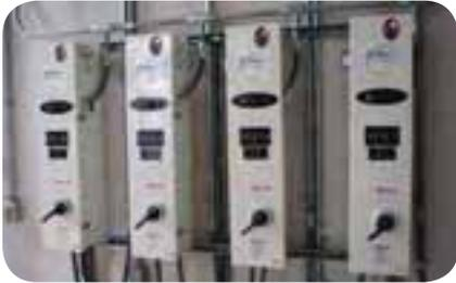
*Variable frequency drive fan controls for Ryerson Base save energy by running motors at less than 100% output when full power isn't needed.*
