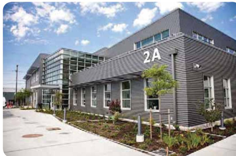
*The LEED Gold certified Atlantic/Central Operations Base includes highly reflective roofing and paving, an exterior vegetated wall that provides shading for the west façade, native vegetation, low-flow water fixtures and natural daylighting.*
