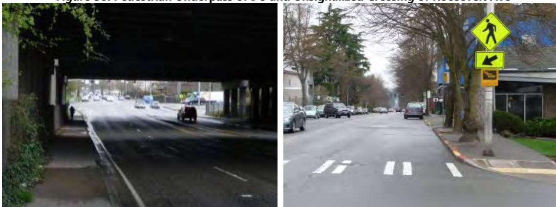
Figure 38: Pedestrian Underpass of I-5 and Unsignalized Crossing of Roosevelt Ave
